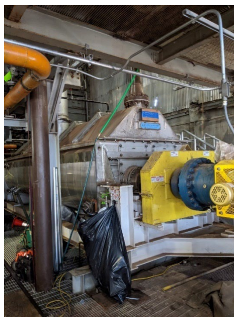
Sludge Dryer in Construction
