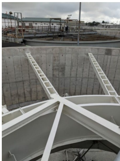
Clarifier 1 Nearing Completion
