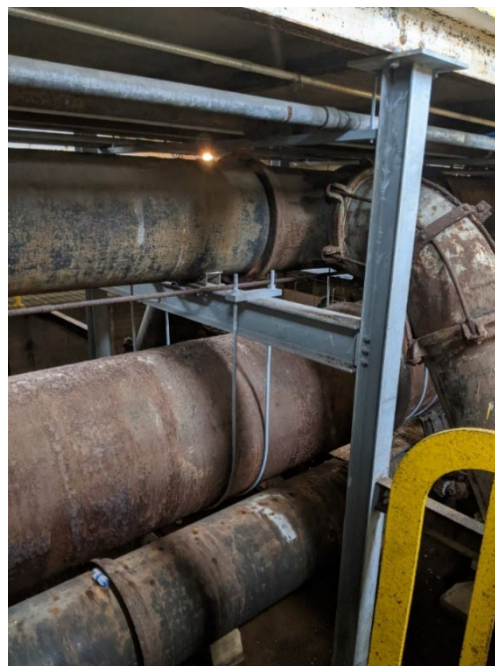
Sycamore Filter Pipe Support Rehab
